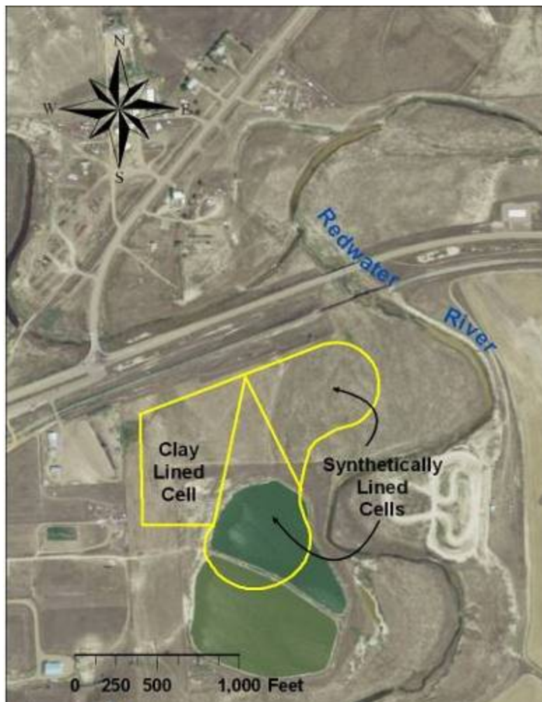
Figure 5-4. Footprint of the newly-constructed Circle wastewater treatment pond system on a pre-construction aerial photograph.
