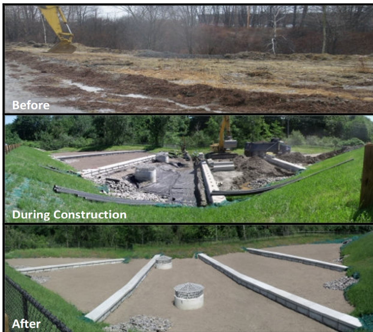
Installation of soil media filter during Mall Plaza Phase. I
