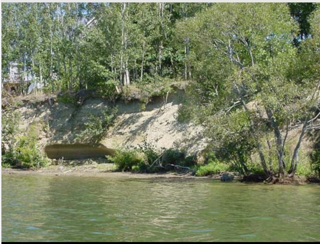
Shoreline erosion along the eastern shore of Sabattus Pond
