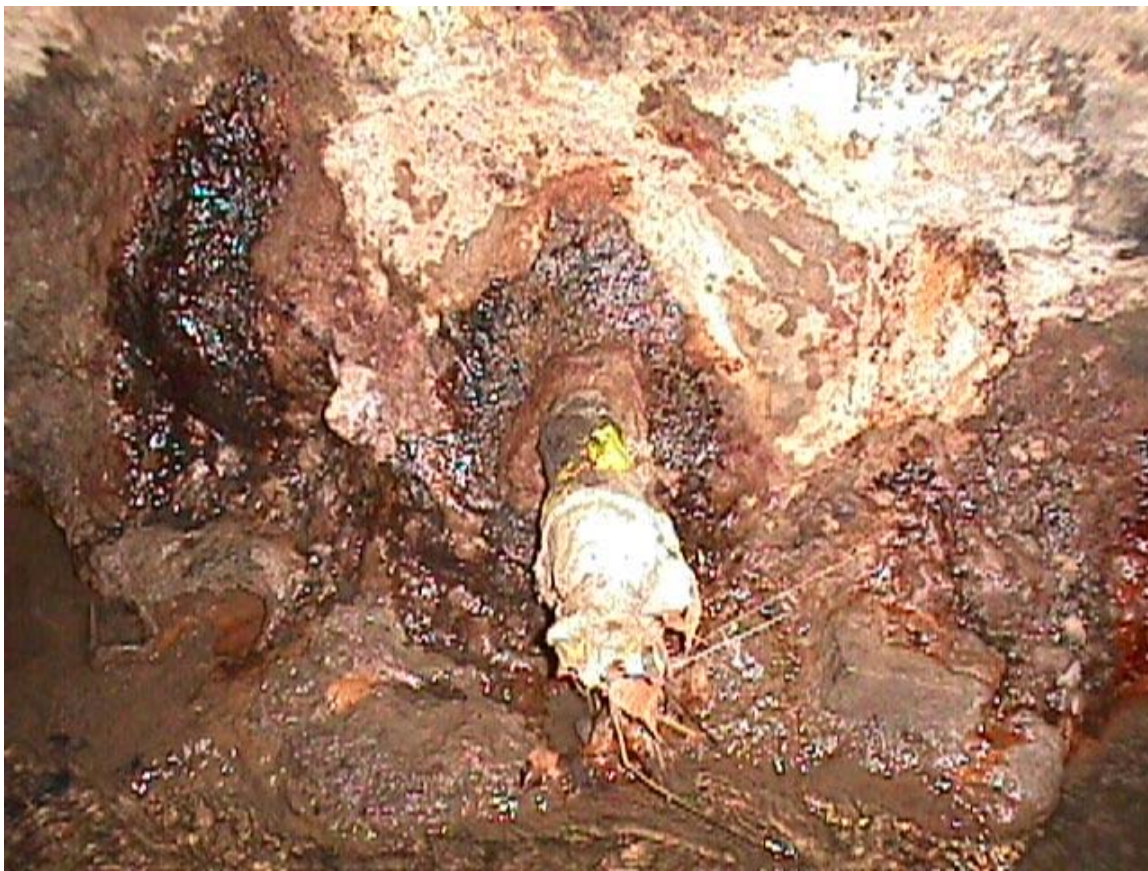
Figure 2.8 Seep located under Greenville Ave. Bridge adjacent to former Beverley Exxon site. Pipe shown in picture is believed to be pipe that was installed to recover gasoline free product from the site. Picture taken 3/2/06.
