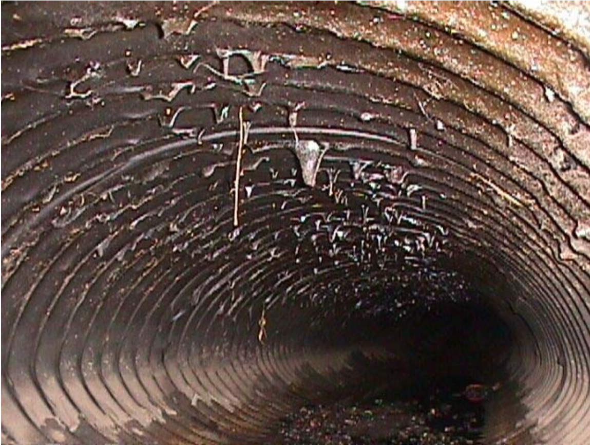
Figure 2.9 Storm drain located under Greenville Ave. Bridge adjacent to former Beverley Exxon site. Tar-like material dripped and hardened from top of storm drain. Picture taken 3/2/06.
