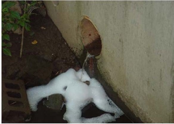
Figure 5.1 Photo of an illicit discharge from a storm sewer outlet.
