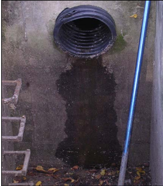
Figure 5.5 Photo of a sanitary sewer overflow pipe in the Walnut Creek Sewer District Leitnaker Road Pump Station. When the pump station becomes hydraulically overloaded, untreated wastewater discharges through the pipe to an unnamed tributary of Pleasantville Creek.
